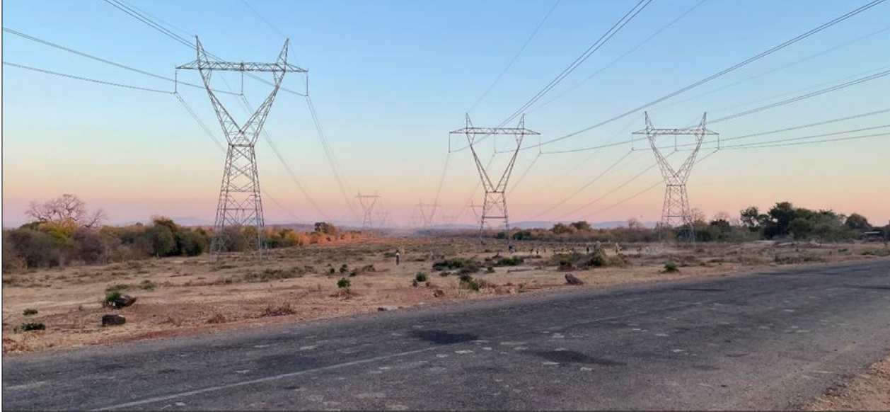
Figure 18-81: 330 kV transmission crossing the D500 just east of the Njame area
