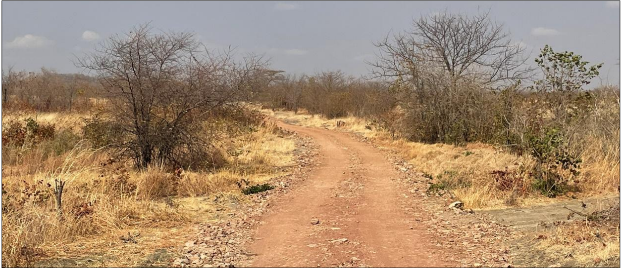
Figure 18-6: view of existing access track from D500 to Hachibozu village (showing recent repairs undertaken by GoviEx) looking south (July 2023)
